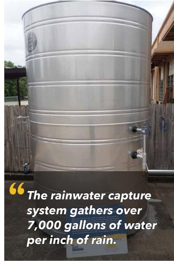
“The rainwater capture system gathers over 7,000 gallons of water per inch of rain.”
